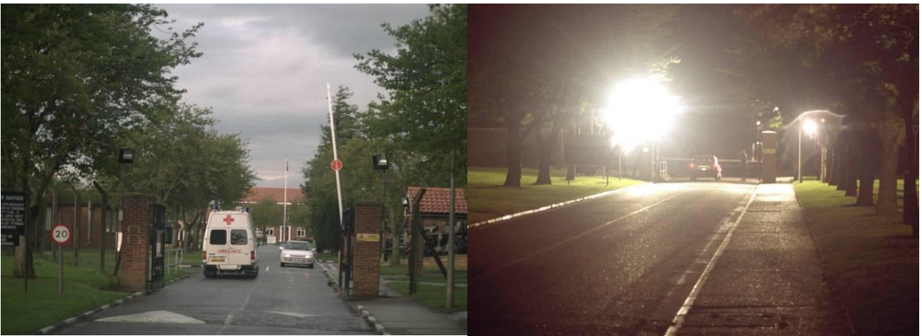
Lighting deployed at a vehicle check point / entrance
