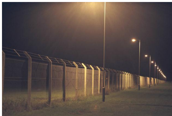
Typical Perimeter Lighting using 100w SON on 8 Metre Columns
