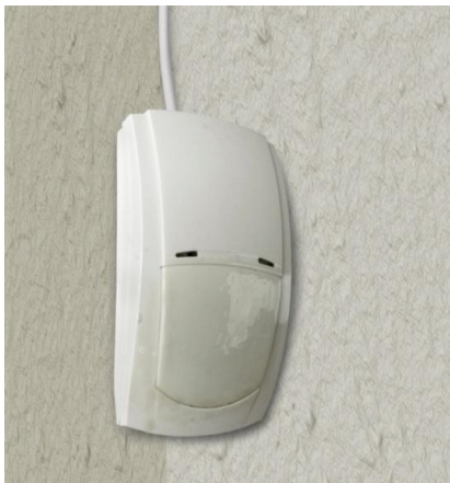
Figure 10: A Detector masked with paint. Examine the detector closely as the presence of some masking materials may not always be obvious.
