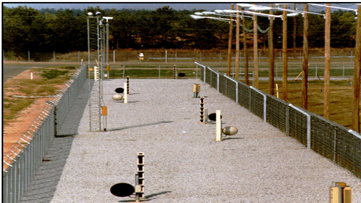
Figure 2-7b: Double Fence Line
