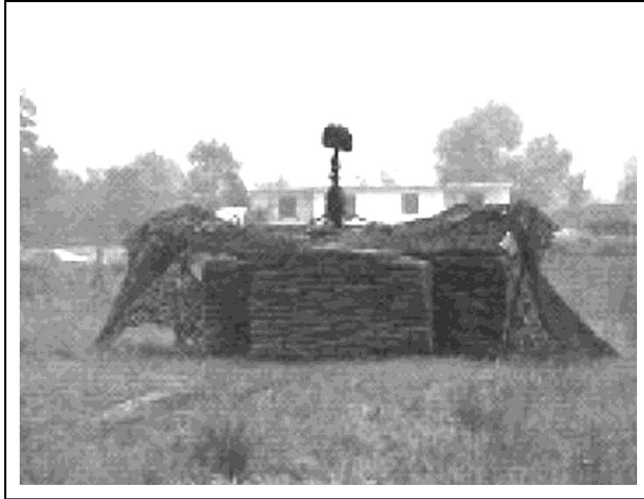
Figure 4-5. Sandbags employed for blast protection
