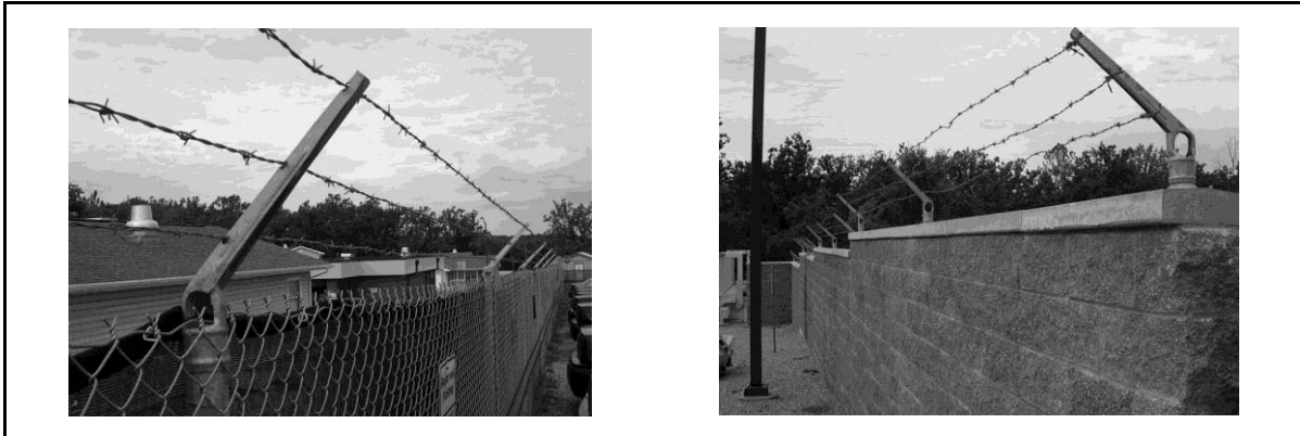
Figure 4-8. Single top guard barbed tape
