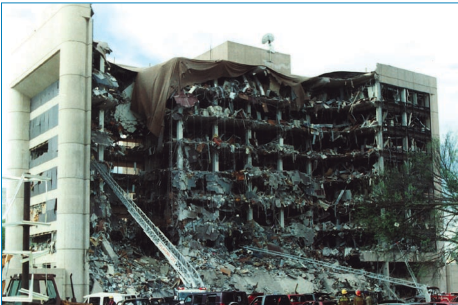
Figure 1-3: The Murrah Federal Building, Oklahoma City 1995.
