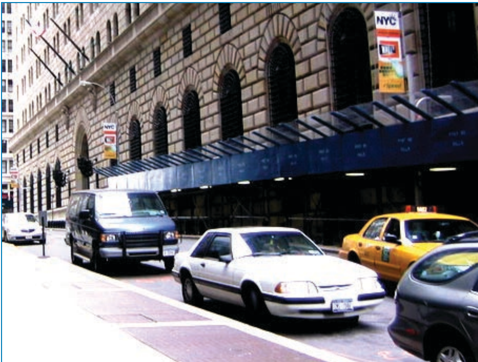
Figure 6-29: Lengthy shelter for curb lane drop-off and pick- up area.
