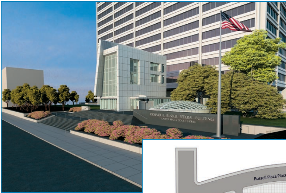
Figure 5-11: Separate screening pavilion for visitors at building entrance. Well-designed structure blends with other site features and maintains character of surrounding context.
