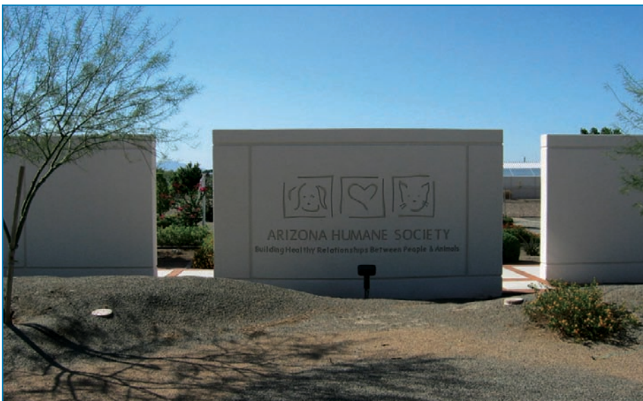
Figure 4-9: Reinforced wall barrier with artwork.
