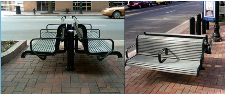
Figure 4-34: Outdoor seating reinforced with hidden bollards.
