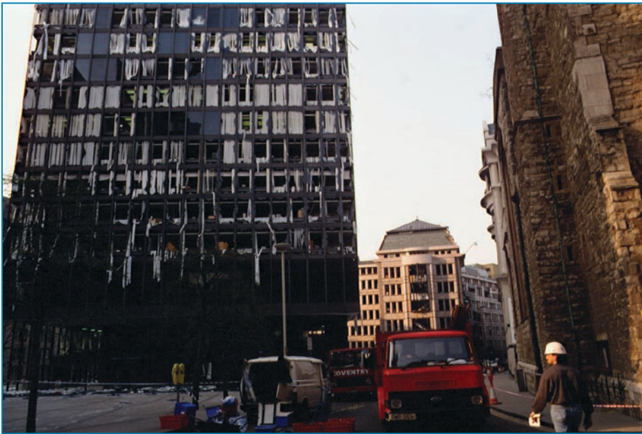
Figure 1-7: Damage to surrounding buildings © MATTHEW POLAK/CORBIS
