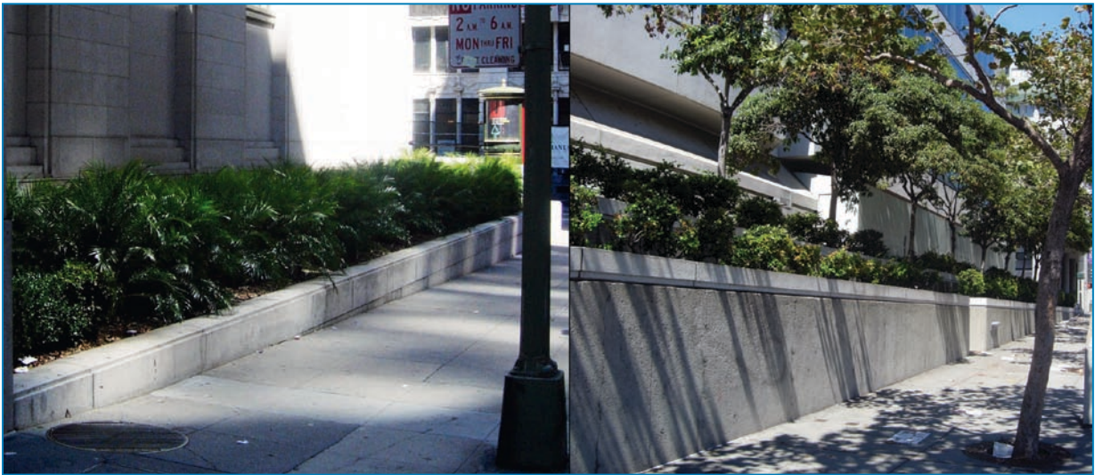
Figure 6-13: A typical raised low planter (left) may be too low to present a significant barrier to vehicles. The high stepped yard (right), which runs along the side of the building, is a significant barrier and could also act as a blast deflector from a curbside vehicle.
